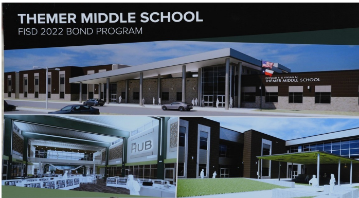
On April 18, 2023, the groundbreaking for the Donald P. & Vivian N. Themer Middle School of Forney happened. The school will open in the fall 2024.
